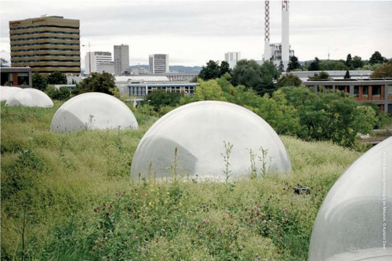
Glass spheres incorporated into the ceilings of spaces, providing the changing views of the sky overhead when indoors, especially for people with limited mobility.
